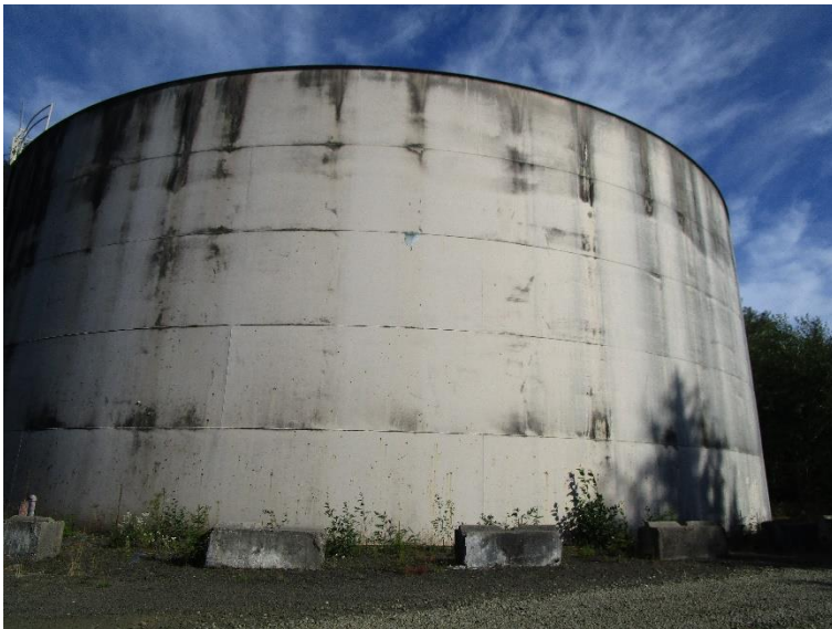
Raymond Heights Reservoir prior to coating application
