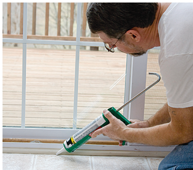
Caulk cracks where roaches hide.
