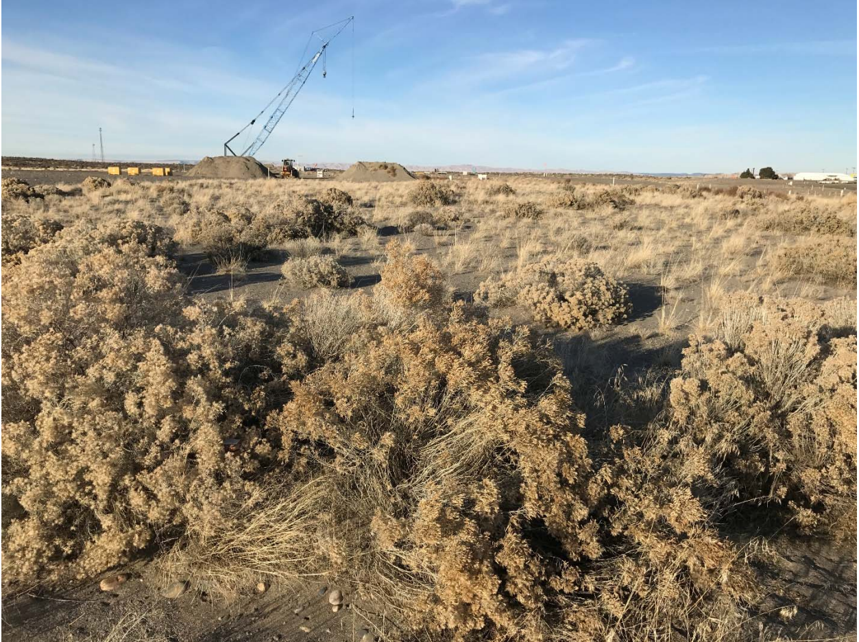
Attachment – Trench 16 in area sampled.
