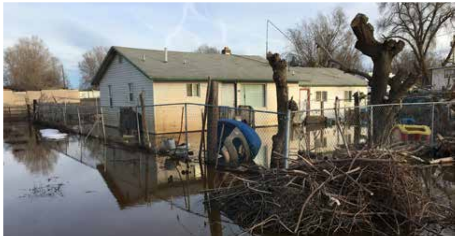
Manure-contaminated floodwater inundated properties, surrounded private wellheads, and damaged four homes. Photo by Ignacio Garcia, WSDA.
